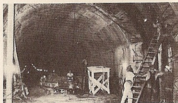
REMOVING last beam from bulkhead at south end of tunnel, showing thick concrete case.
