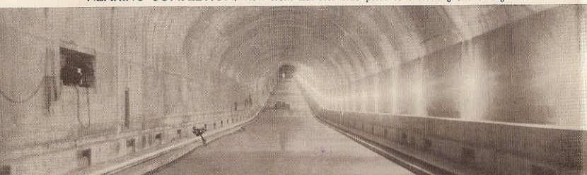
NEARING COMPLETION, view from LaPorte side prior to installing tile lining.
