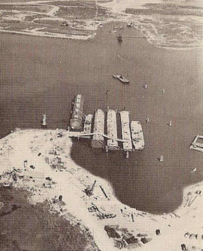
LOOKING NORTH toward Baytown and approach road across Black Duck Bay, with steel tubes in various stages of receiving concrete coating.
