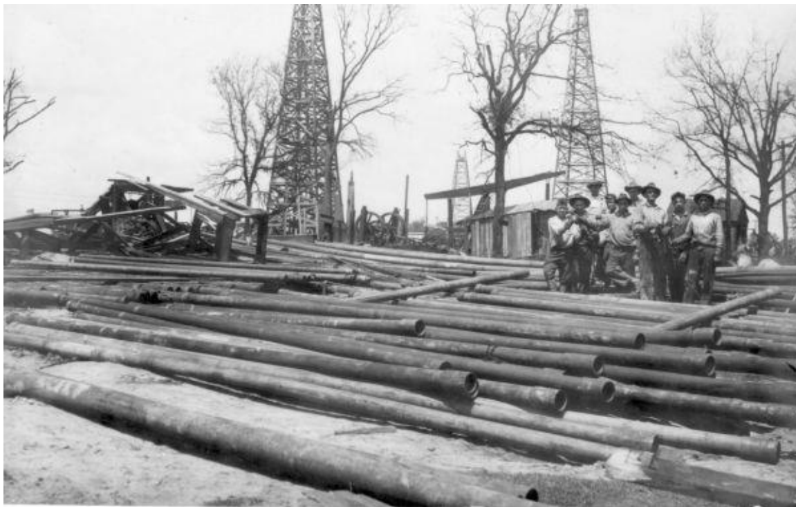
Image 5. This photograph, probably taken after the 1919 cyclone or 1921 hurricane, shows a walking beam and bull wheel in the background. The walking beam served as a pump jack to extract oil from wells which had stopped flowing. They did not have the characteristic “donkey head” shape of modern pump jacks. Texas Energy Museum.
