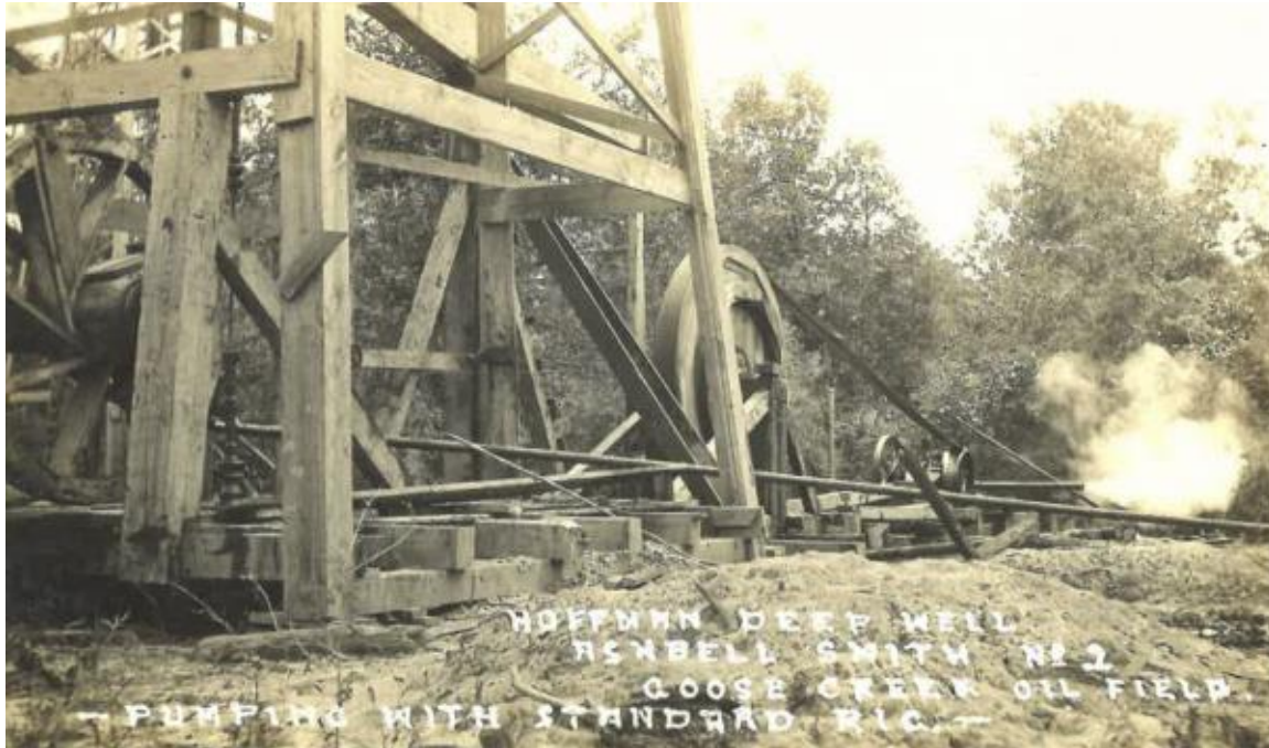
Image 4. The Standard Rig , also known as a cable tool rig, was still being used years after rotary drilling started and even after the Hughes cone bit hit the market. Here, it is used to pump a finished well. This picture was probably taken in late 1916. Courtesy Jeff Spencer.
